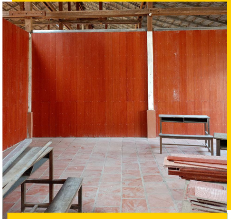
The new partition walls are being installed
